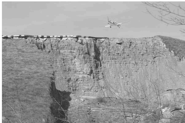
FIGURE 13. Five years after its construction, collapse of a large reinforced soil structure at Yeager Airport, WV, destroyed the community below.
