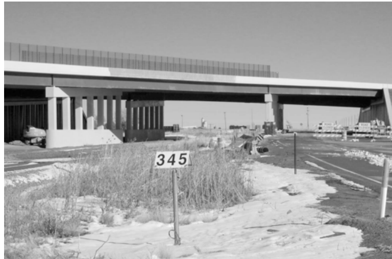
FIGURE 10. New triple-span bridge on I-70 over the transcontinental railroad near Denver's airport. The east end (right) is supported by reinforced soil. Pipeline marker is in foreground.
